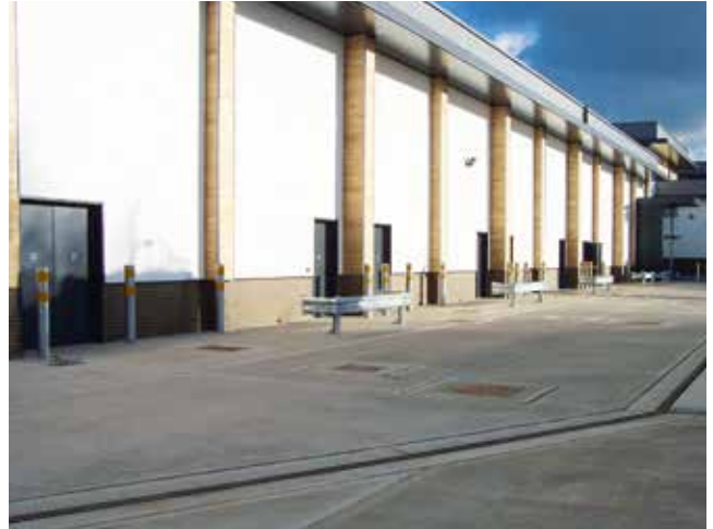
Installation in concrete surface
