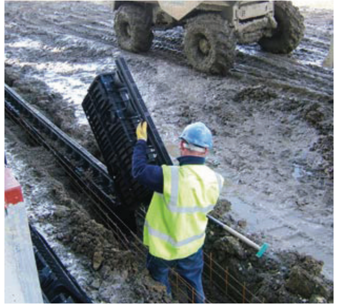
Lightweight elements, installed by one single worker.
