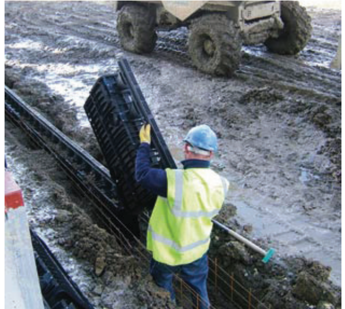
Lightweight elements, installed by one single worker.
